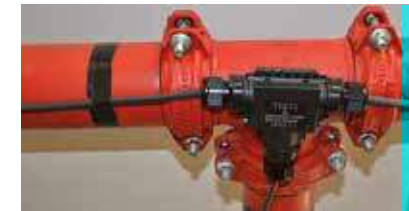
Connection of heating cables (France). Series TH211.
